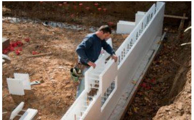
FIGURE 24 – INSULATING CONCRETE FORMWORK TECHNIQUE
