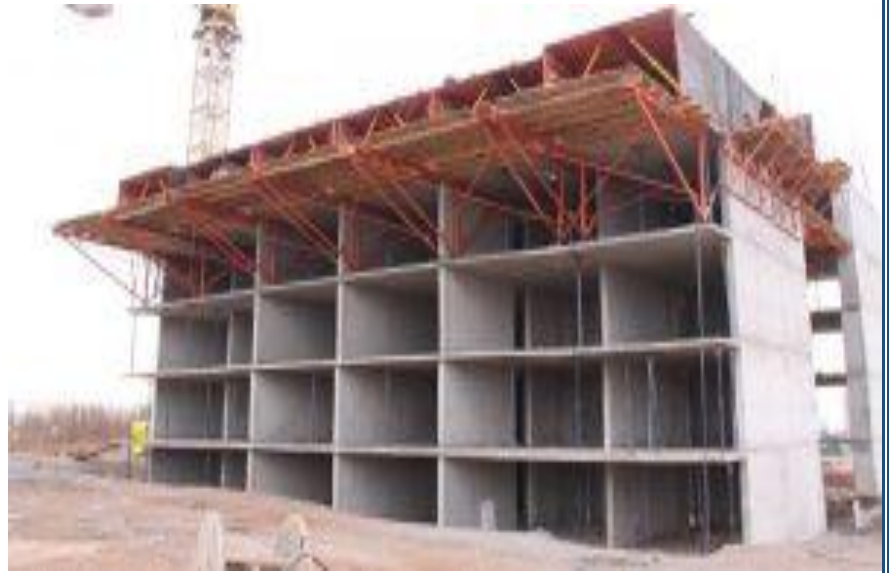
FIGURE 19 - TUNNEL FORMWORK SYSTEM
