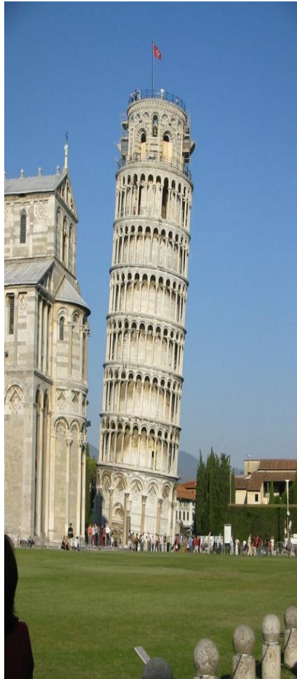
Figure 47 – SOIL FAILURE
